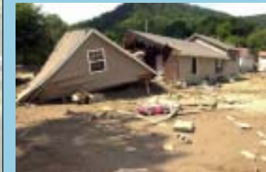
Clear Fork Road, WV, July 14, 2001 -- This house was torn apart by the flooding of the nearby Clear Fork Creek. Photo by Leif Skoogfors/ FEMA News Photo
